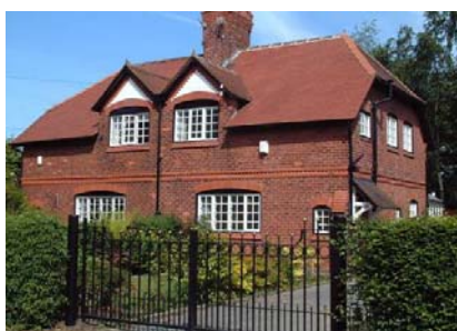
Houses in Rawstorne Road, Penwortham
